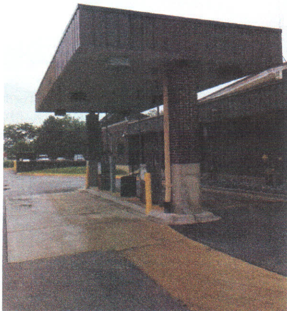
Fuel island (downspout in foreground). Drain from roof leaked and requires replacement.
