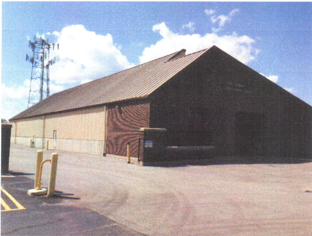
Garage exterior depicting steep roof angles
