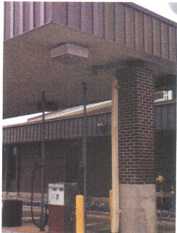
Fuel island (downspout in foreground). Drain from roof leaked and requires replacement.
