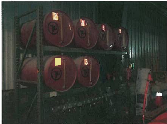
Fluid Storage and Dispensing Rack
