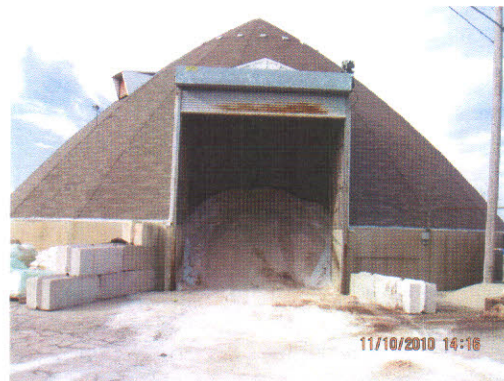
Salt Storage Dome
