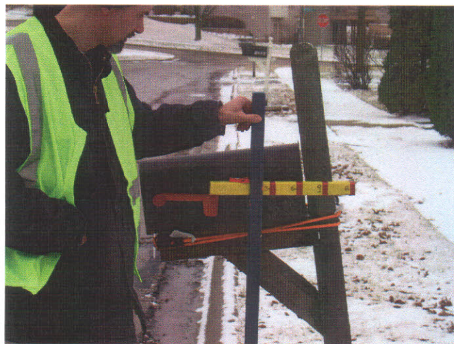
Improperly Installed Mailbox
