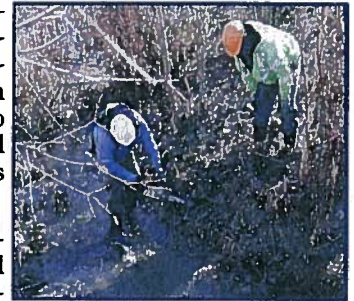
Contractor removes scrub tree obstruction.
