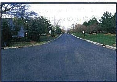
Completed West Street improvements looking north.
