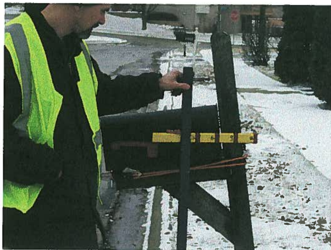
Improperly Installed Mailbox
