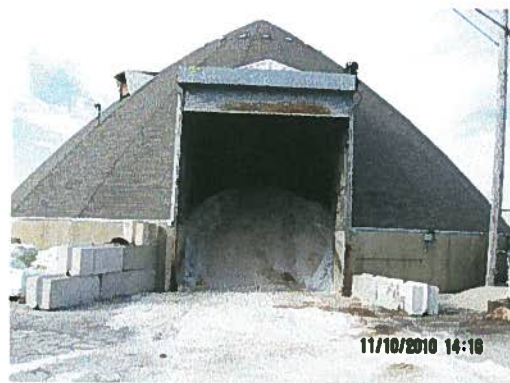
Salt Storage Dome
