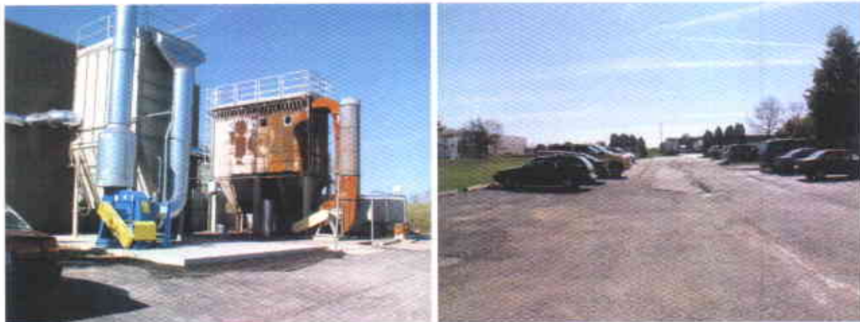
DUST COLLECTION EQUIPMENT AND PARKING LOT PAVEMENT AT 457 ST. PAUL
