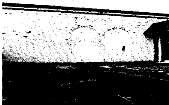
WALL FACING NORTH AVENUE
