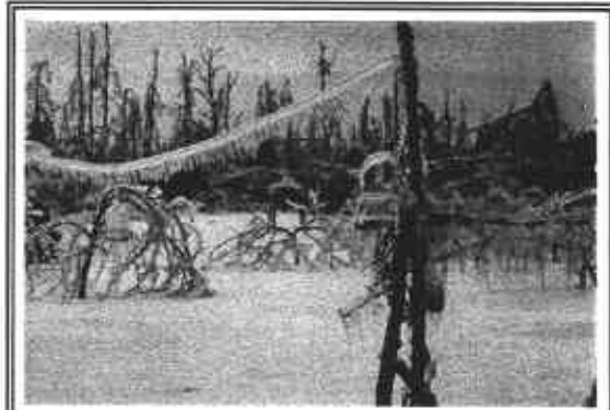
Above ground lines are especially susceptible to damage by ice storms. The loss of power has a ripple affect to many other properties.
