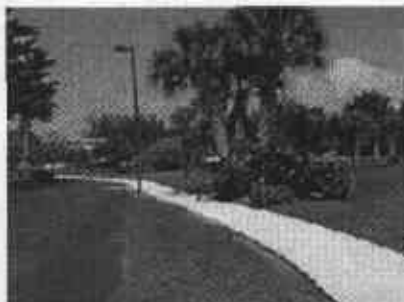
In April 2003, Full Circle provided Goodlette Arms residents with 200+ yards of new sidewalk. The sidewalk provides residents with a safer route to Goodlette Road, and more room to get out and enjoy the wonderful Southwest Florida weather.
