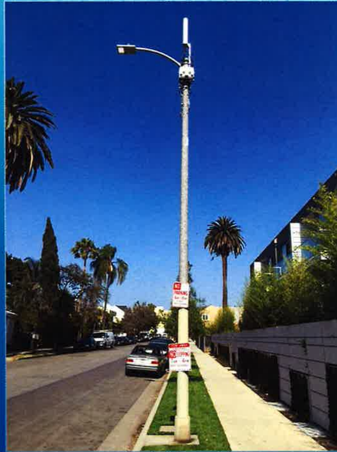
Attachment to a Streetlight
