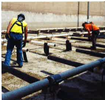
Diffuser replacement in aeration basins.
