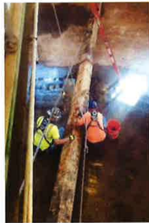
Clarifier sweep replacement.
