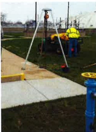
Valve stem replacement.
