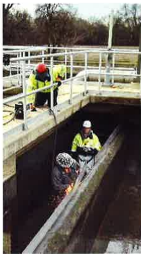
Replacement of final weir on aeration basin.
