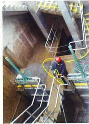
Influent screw pump pit cleaning.
