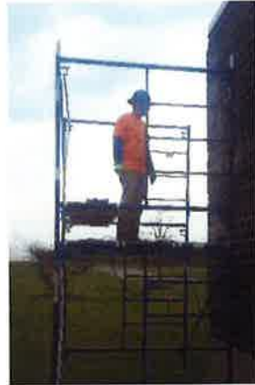
Tuck-pointing the brick on the sand filter building.
