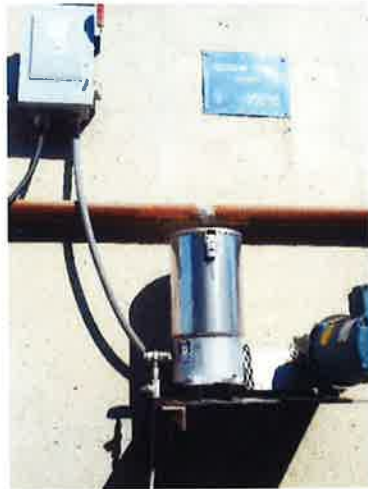
Replacement of grease pump unit.
