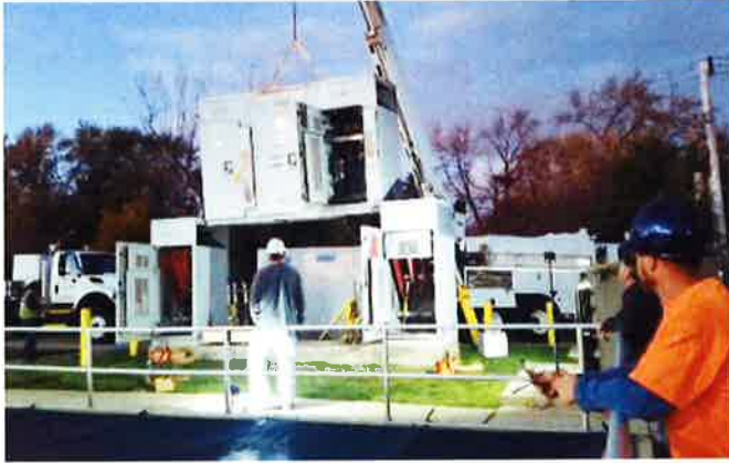
Replacing the ComEd ATO using a large crane.
