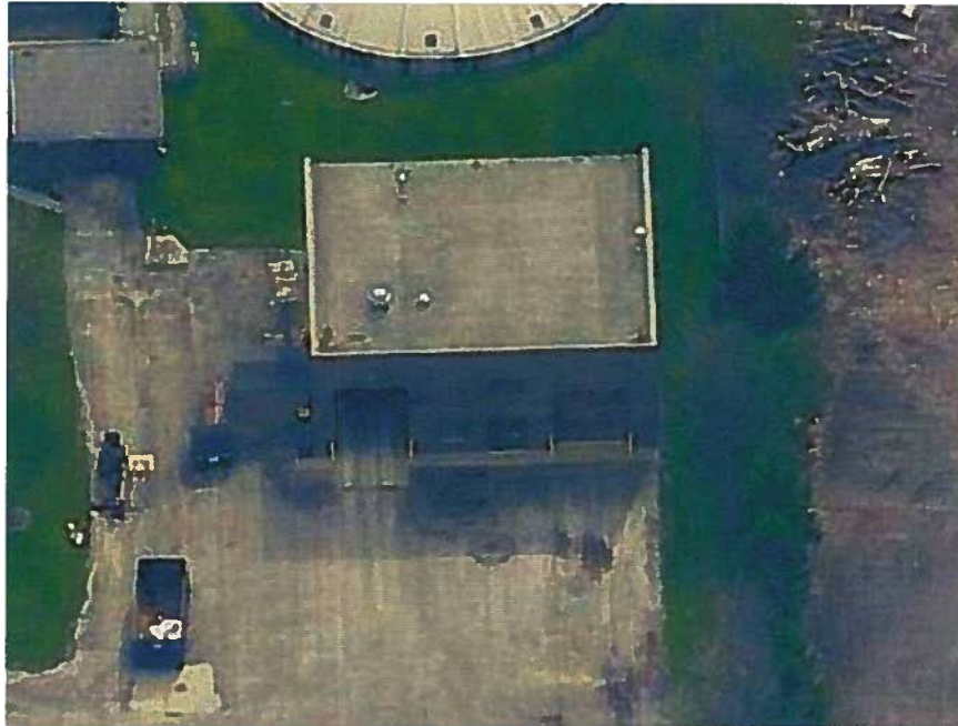
Replaced WRC Sludge Building Roof
