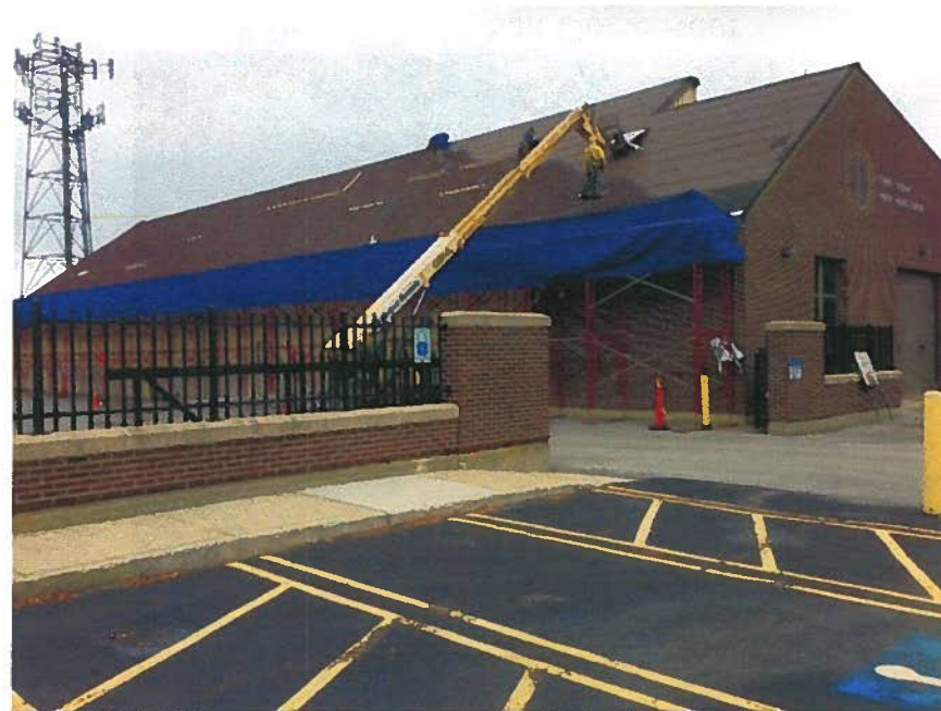
PWC North Garage Roof Being Replaced
