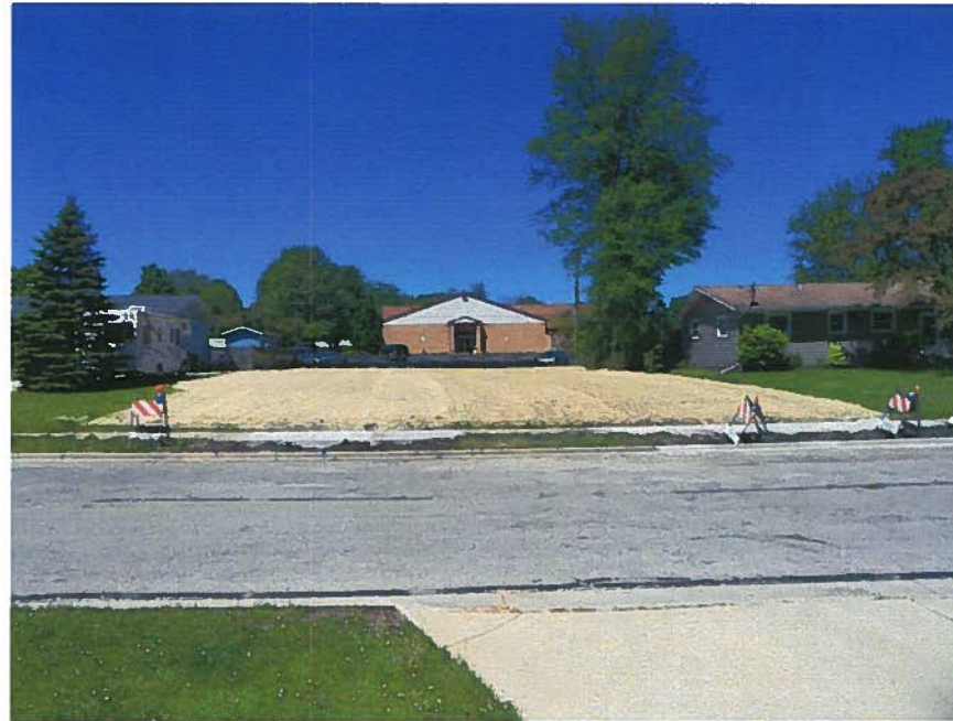
Razed Flood Prone Structure & Restored Lot
