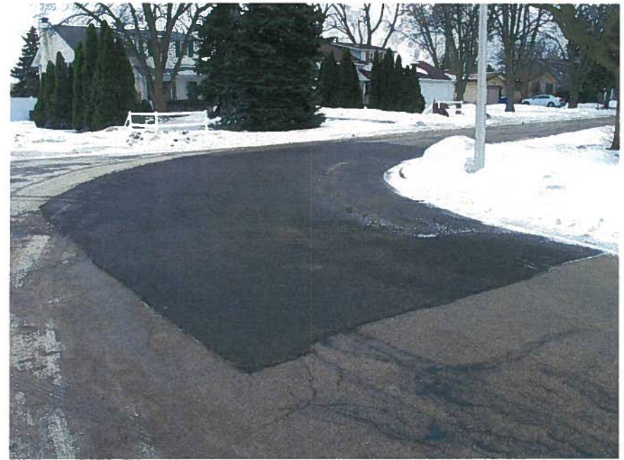
Pavement Patch at Inca Boulevard & Arrowhead Trail
