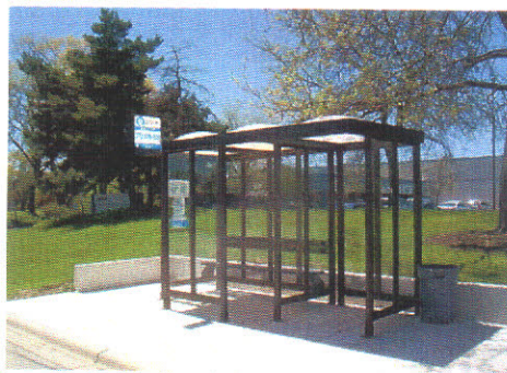
This non-ad shelter design is prevalent in many communities in northeastern Illinois.
