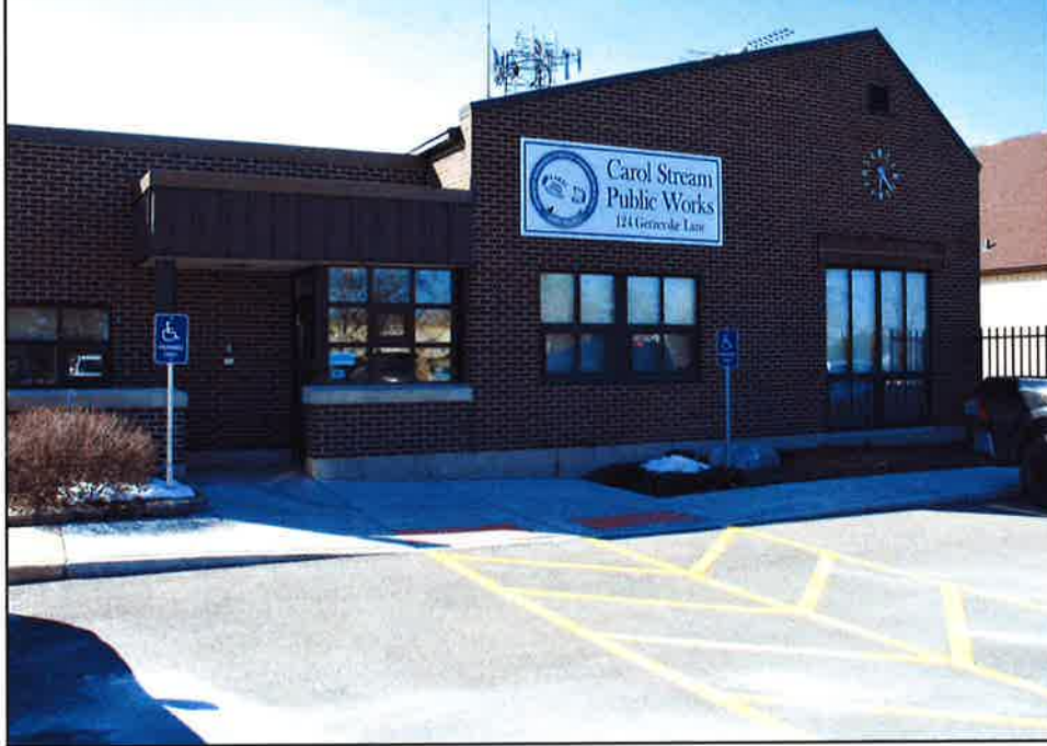
PWC Admin. Building Roof Replacement Project
