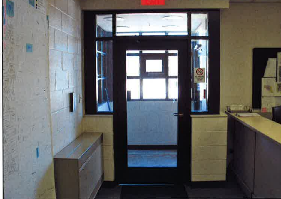
PWC Admin. Building ADA & Security Improvements Project
