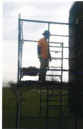
Tuck-pointing the brick on the sand filter building.
