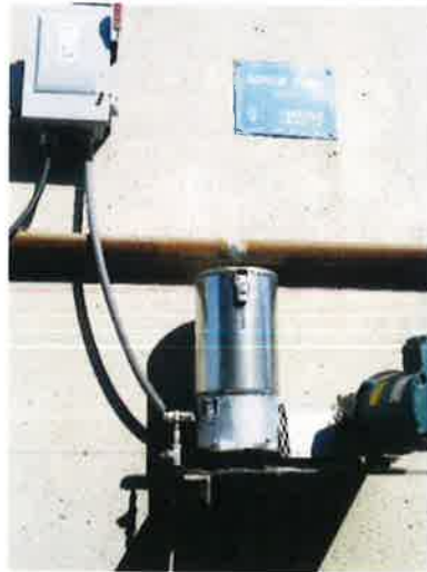
Replacement of grease pump unit.
