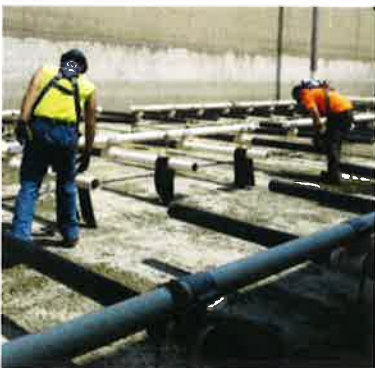
Diffuser replacement in aeration basins.
