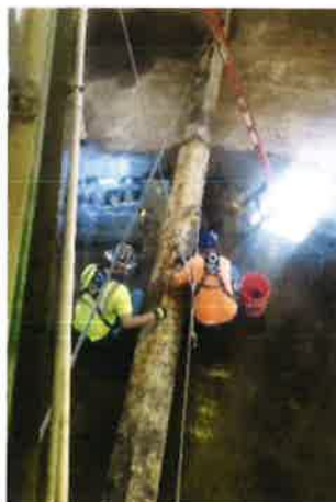
Clarifier sweep replacement.
