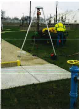
Valve stem replacement.
