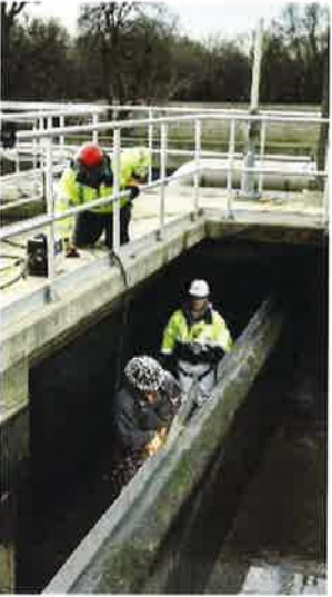
Replacement of final weir on aeration basin.
