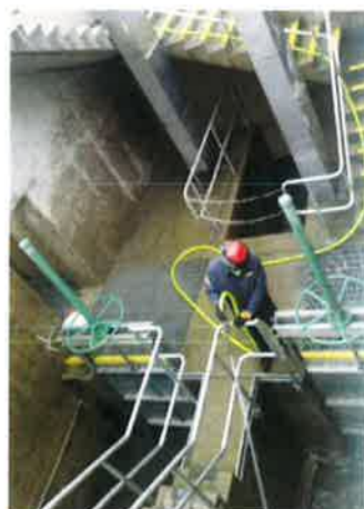
Influent screw pump pit cleaning.
