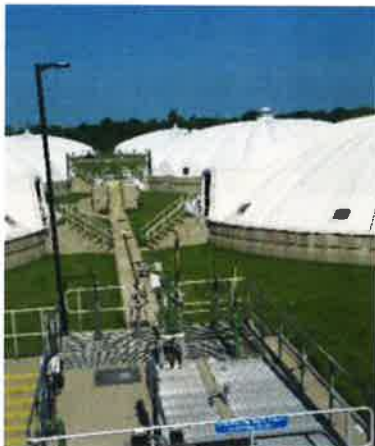
New LED light poles and fixtures.
