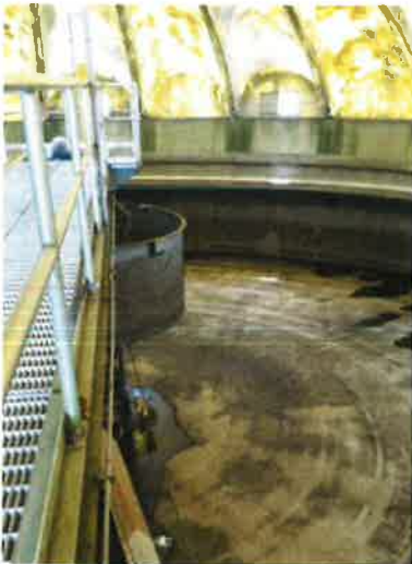
Replaced wear strips and ball bearings on the main gear at clarifier #2.
