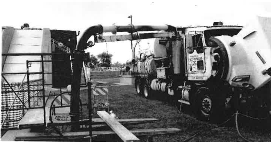
Valve vault installation at influent drain valve.
