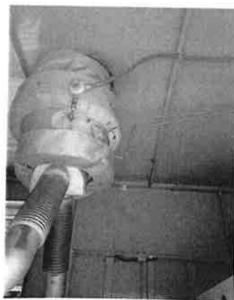
Catalytic converter and controls installed on generator.
