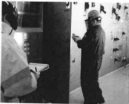
Completing infrared imaging on an electrical panel.
