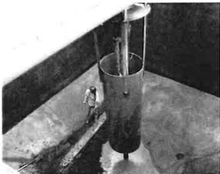
Repairing grit tank inductor.
