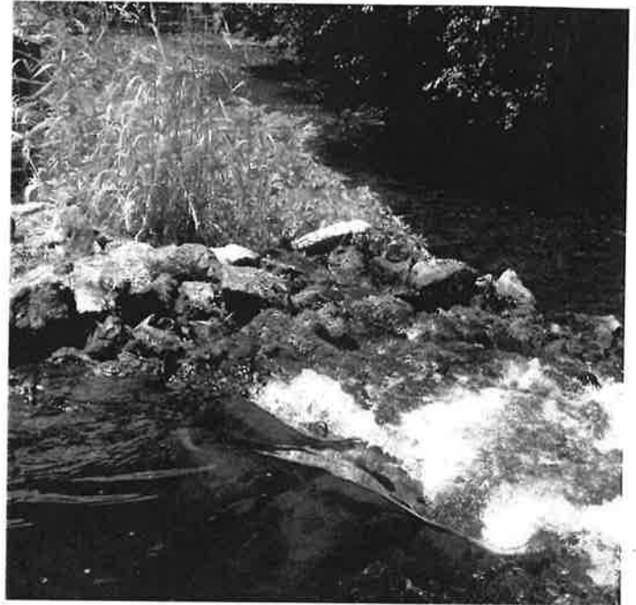
Finished treated effluent into Klein Creek.
