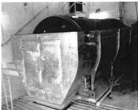
Rehabilitation of the Hycor units.
