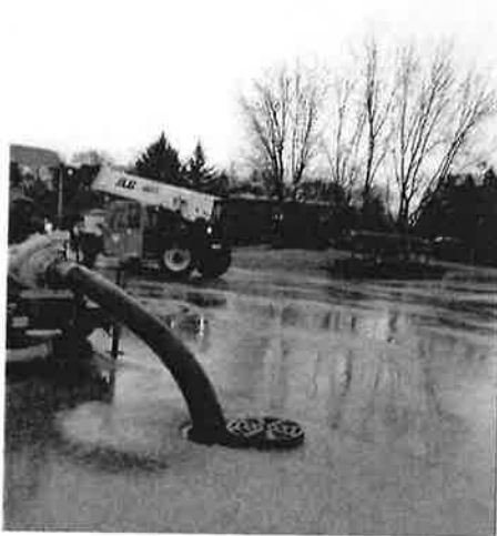
Emergency bypass pumping standing by during primary screw pump repairs during rain event.
