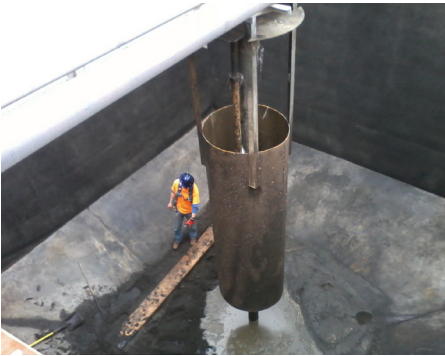
Repairing grit tank inductor.
