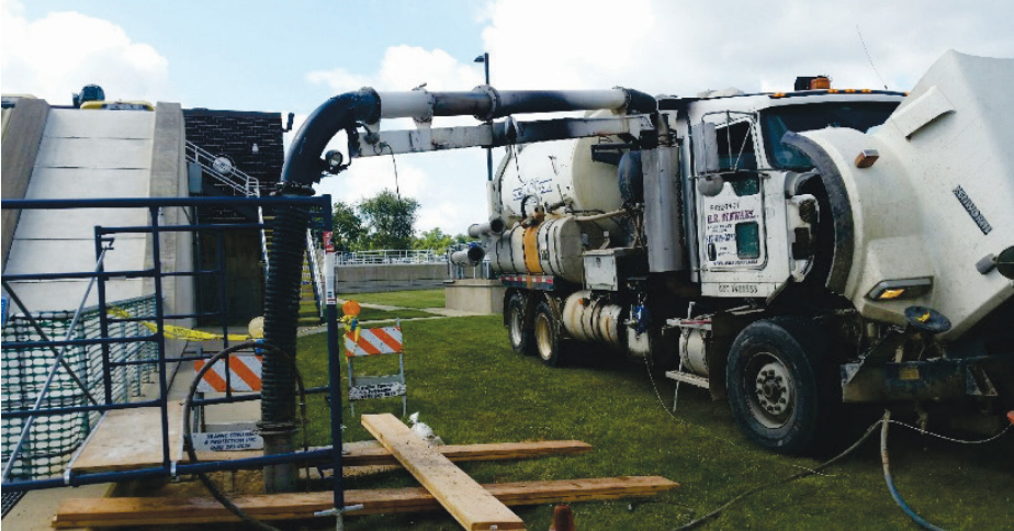
Valve vault installation at influent drain valve.
