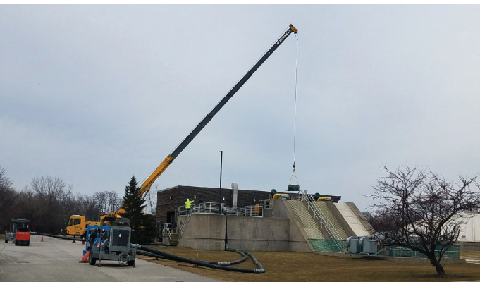
Primary screw pump repairs, coupling, motor, and gearbox replacement.
