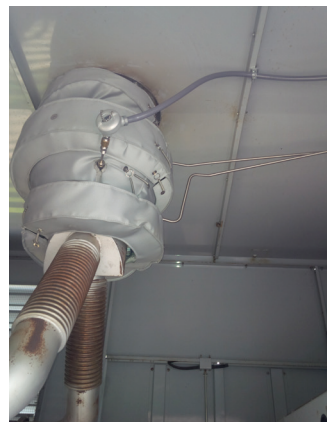
Catalytic converter and controls installed on generator.
