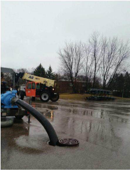
Emergency bypass pumping standing by during primary screw pump repairs during rain event.
