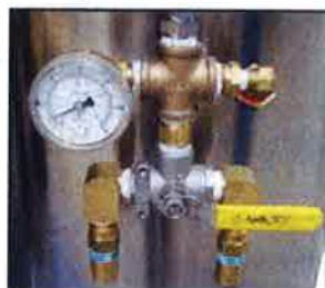
Dual Relief Valve Assembly
