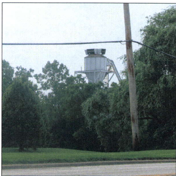
View of existing baler from southbound Gary Avenue
