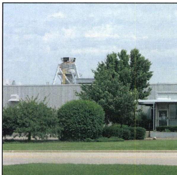
View of existing baler from westbound Fullerton Avenue
