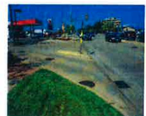
Pipe bursting was designed for the sewer crossing of Dundee Road.
