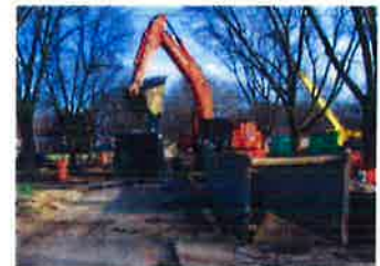
Interceptor construction was through established residential neighborhoods.
