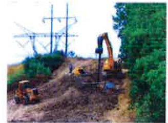
Steep slopes required unique design and construction.
