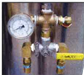
Dual Relief Valve Assembly
