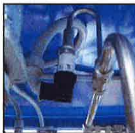
Integrated Bulk Tank Pressure Sensor
