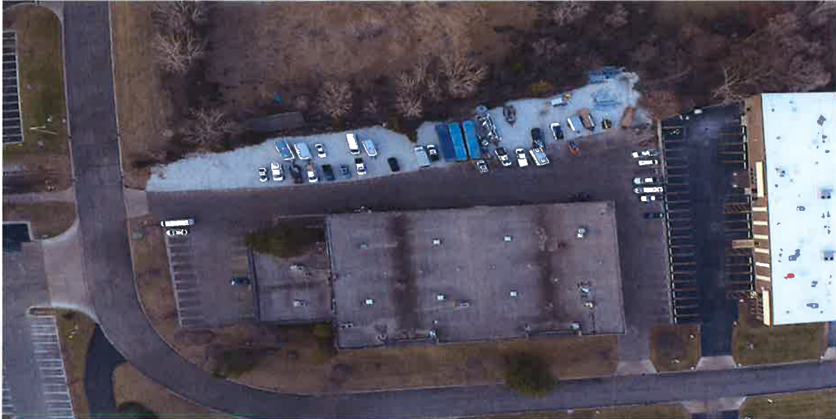
Photos 2: Southern Strip Improvements
