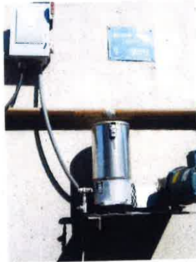
Replacement of grease pump unit.
