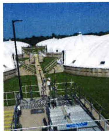
New LED light poles and fixtures.
