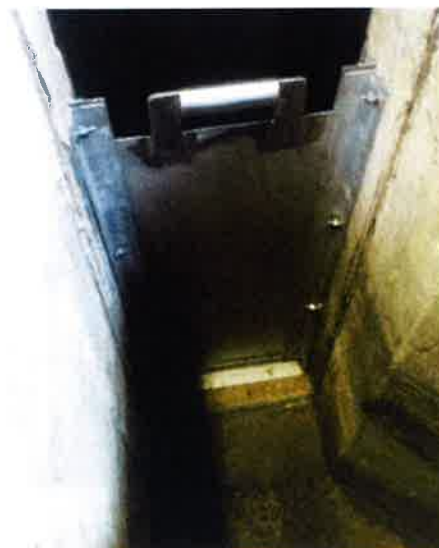
Fabrication of stainless sand filter gates and weirs.
