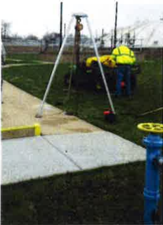
Valve stem replacement.
