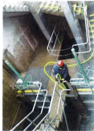
Influent screw pump pit cleaning.
