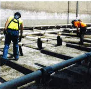
Diffuser replacement in aeration basins.
