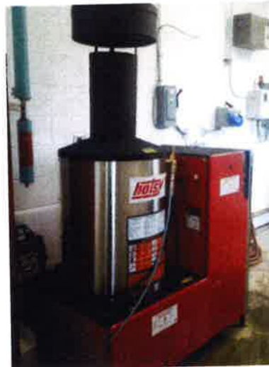
Replacement of steam cleaner.
