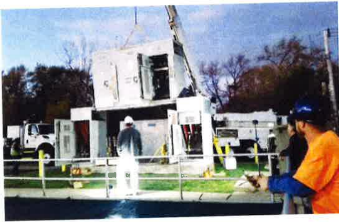
Replacing the ComEd ATO using a large crane.
