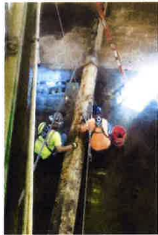
Clarifier sweep replacement.
