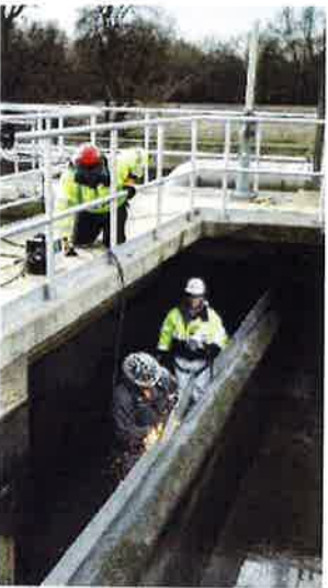
Replacement of final weir on aeration basin.
