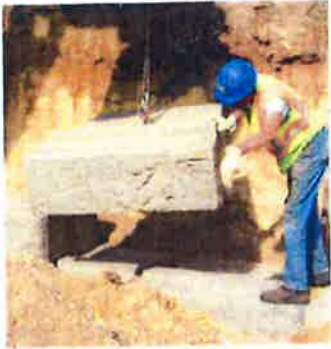
A block being set in place with a backhoe and chain.
