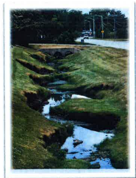
Figure 2 - Section I; Looking West
