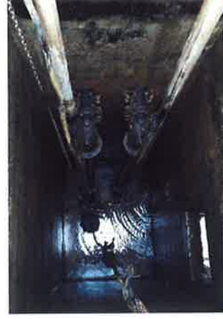
Repairing the pump.
