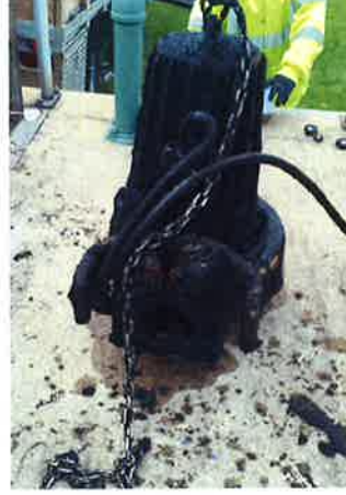
Repairing the waste activated sludge (WAS) pump.
