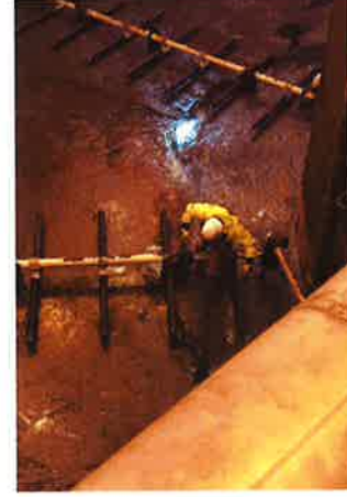
Making repairs in the digester.
