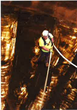
Working in clarifier.
