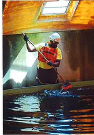
Working in clarifier.
