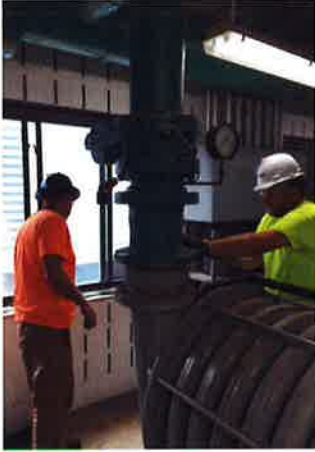
Repairing the blower leaks.
