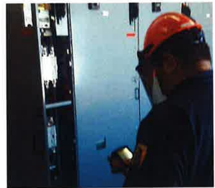
Infrared imaging of electrical panels.
