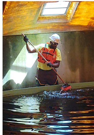
Working in clarifier.
