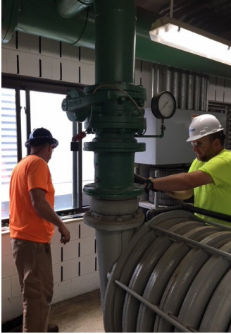
Repairing the blower leaks.
