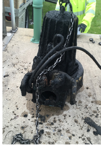
Repairing the waste activated sludge (WAS) pump.
