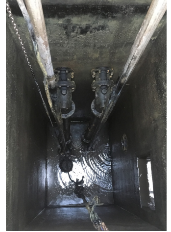
Repairing the pump.
