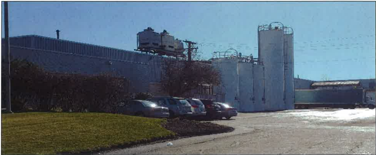
Photo of Existing Silos on West Side of Property
