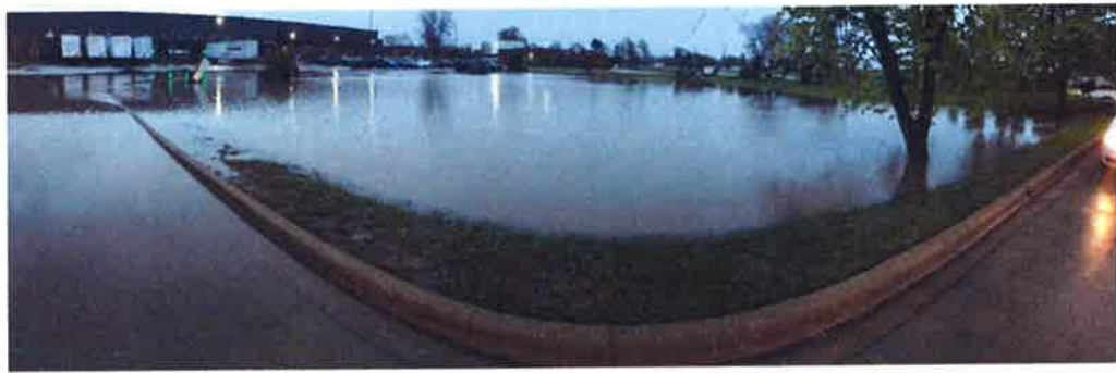
East Pond (285 E Fullerton Ave) during 05/15/20 rainfall.
