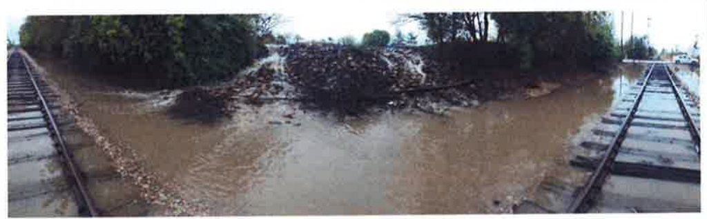
Overtopping of Emergency Spillway during 05/15/20 rainfall.
