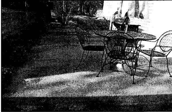
Existing concrete patio in rear yard. Note retaining wall on neighbor's property and significant grade change between properties.
