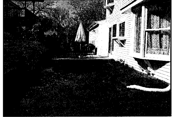
Another view of existing concrete patio in rear yard and the retaining wall near the property line between the two properties.
