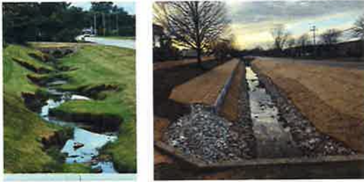
$85K Water Quality Improvement Program from DuPage County
