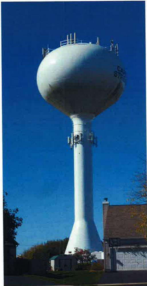
1 OVERALL TOWER PHOTO SCALE: N.T.S.
