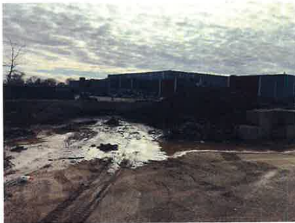
Spoil dumping/storage area
