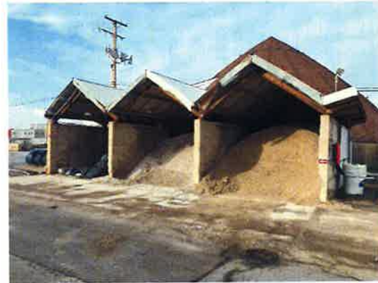
Material storage bins
