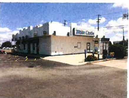
3 - EXISTING EXTERIOR - FOR REFERENCE ONLY
