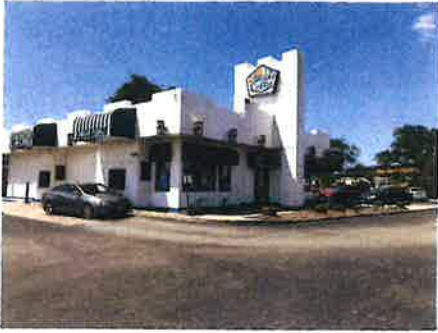
2 - EXISTING EXTERIOR - FOR REFERENCE ONLY
