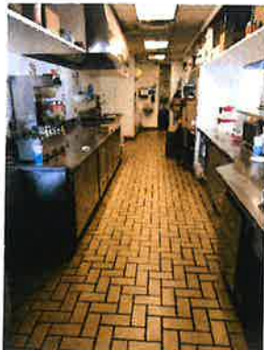
7 - EXISTING INTERIOR KITCHEN - FOR REFERENCE ONLY
