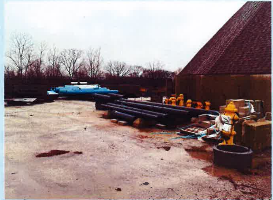
Water/sewer structures to be stored in sheltered area
