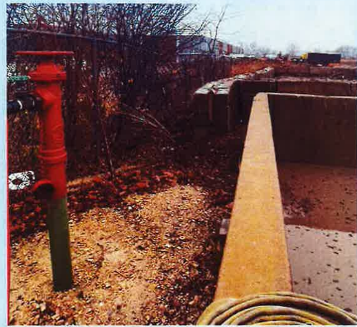
Fence and fence line grading improvements
