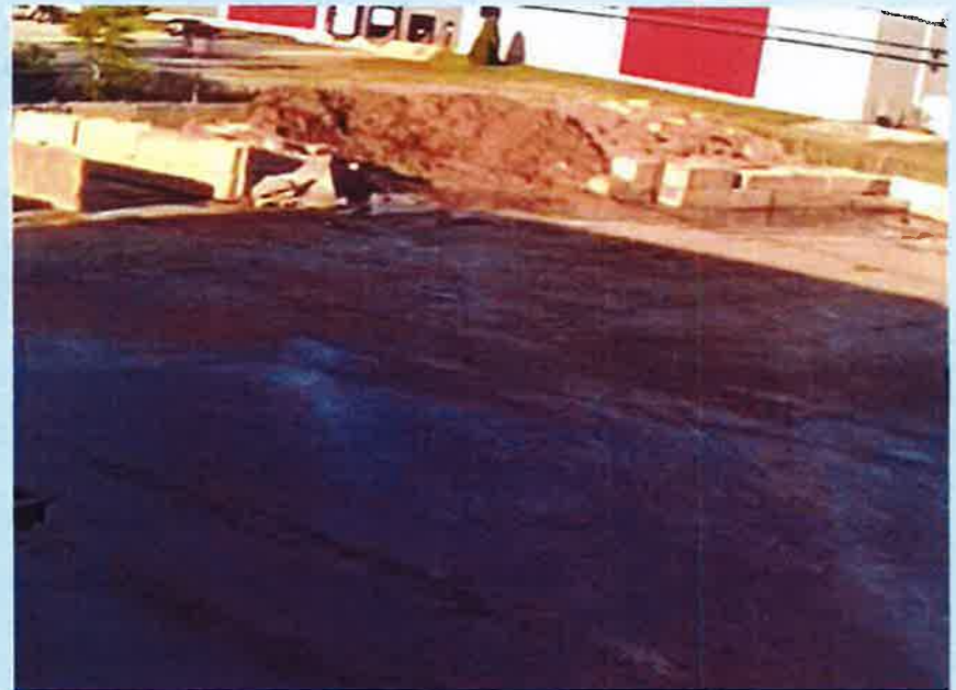
Spoil Separation and Management Area
