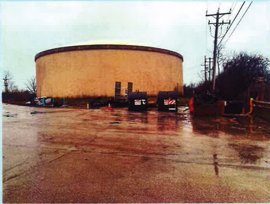
Scrap and trailer storage areas redesigned and paved
