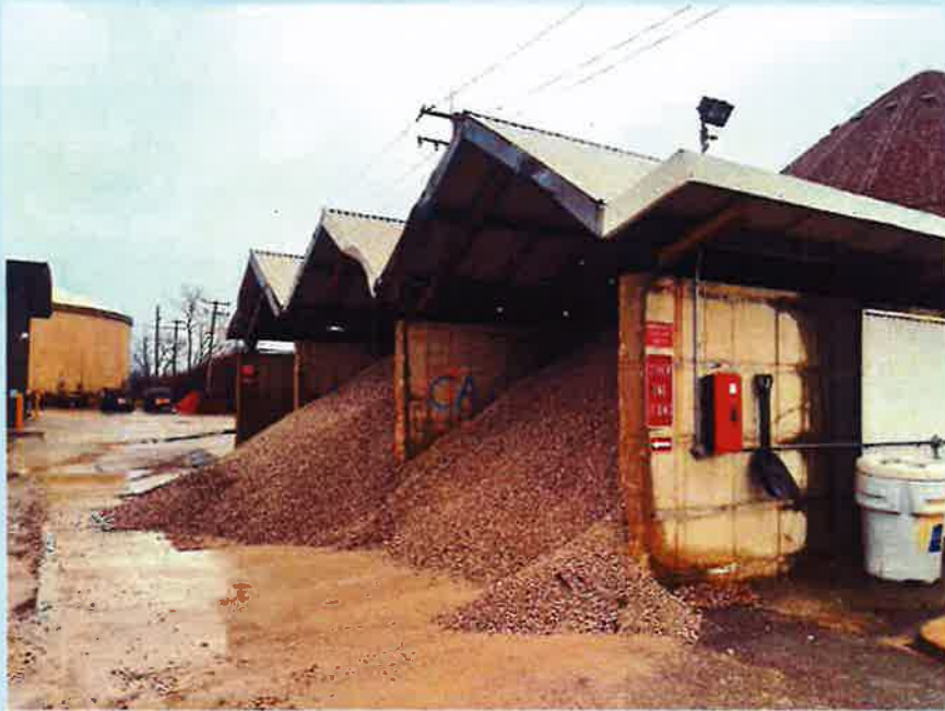
Material storage bins to be re-purposed (plow storage)
