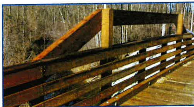
WHEELER TIMBER RECREATION BRIDGES
