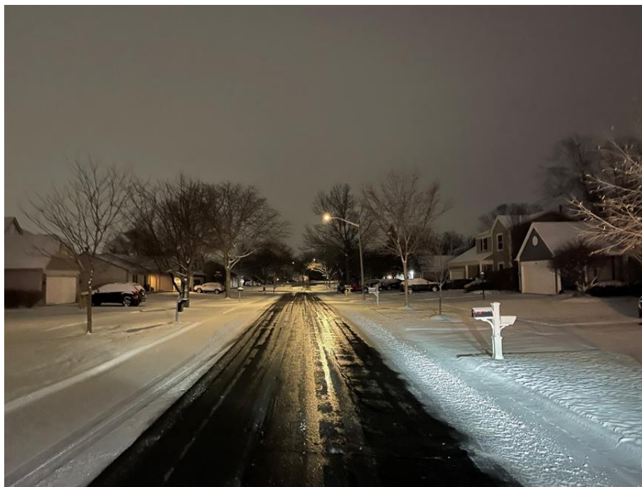
Liquid-only de-icing in residential area
