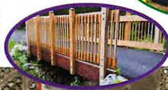
Replace Existing Bridge w/ New Pedestrian-style Bridge Above the Flood Elevation
