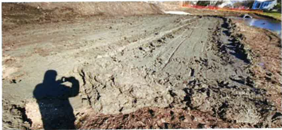
Photo 12 - Unsuitable material from Wall "C" disposed of in Mitchell Lakes (March 16, 2024)
