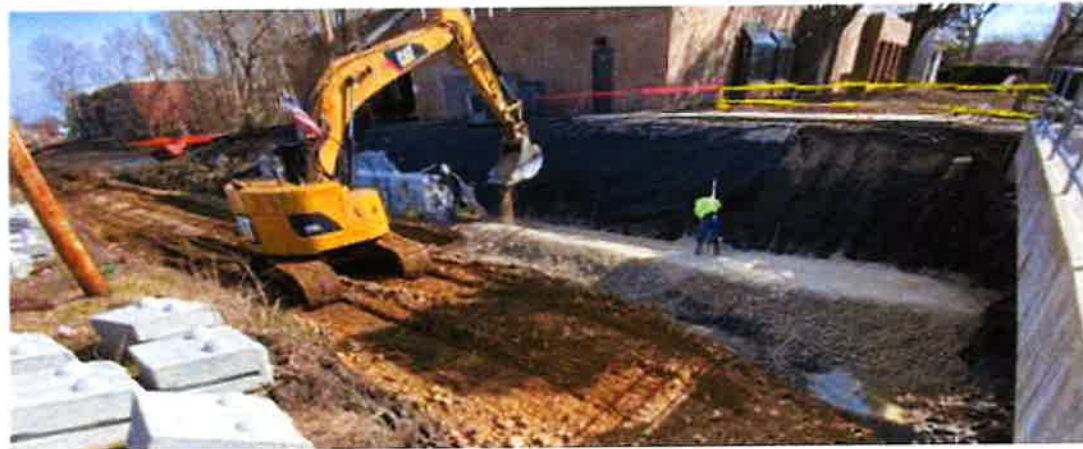
Photo 13 - Final subgrade for Wall "C" created from crushed aggregate (March 16, 2024)
