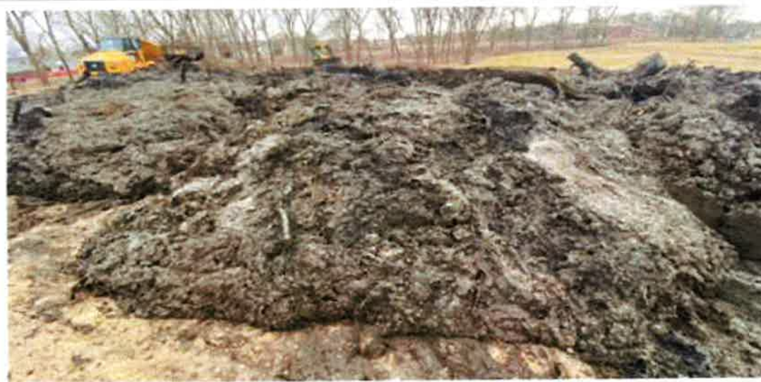
Photo 6 - Unsuitable streambed material being hauled to sled hill (March 4, 2024)
