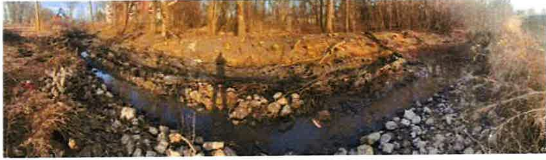
Photo 4 - Ruts in existing streambed caused by tree clearing equipment (February 22, 2024)
