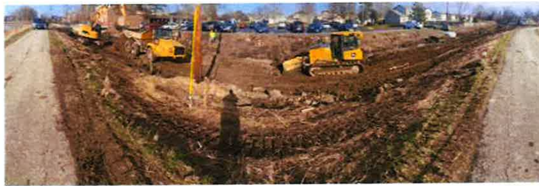
Photo 17 - Backfilling and shaping the streambed using suitable material (March 28, 2024)
