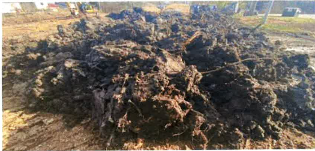
Photo 16 - Unsuitable streambed material being staged before hauling to Mitchell Lakes (March 28, 2024)
