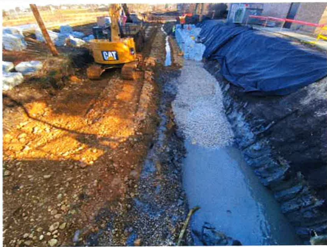
Photo 11 - Backfilling with crushed aggregate after removing the unsuitable subgrade (March 16, 2024)
