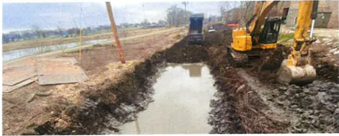
Photo 7 - Suitable material being backfilled into the undercut areas (March 4, 2024)
