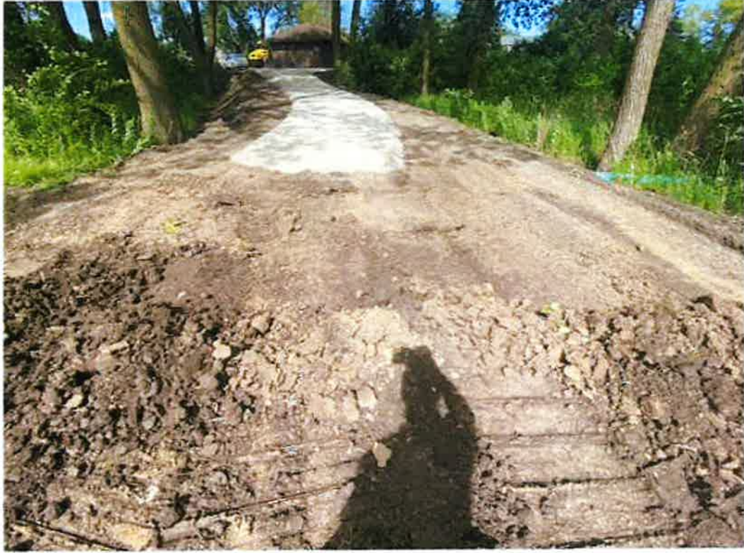
Photo 3 – Looking east after stone was added to the haul route used to construct the sled hill (06.07.2024)
