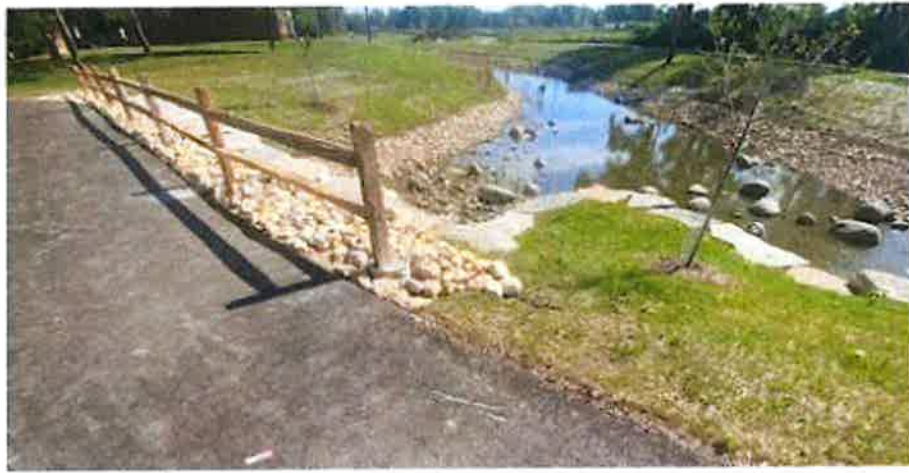
Photo 1 - Mitchell Lakes Outfall
