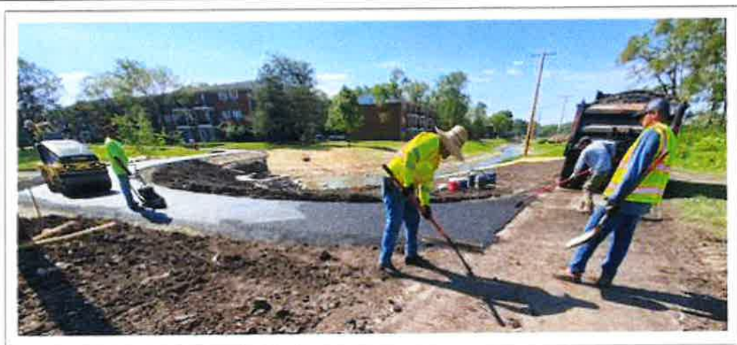
Photo 6 - Looking southeast at the new path over the Mitchell Lakes outfall (06/13/24)
