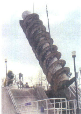
Secondary screw pump rehabilitation.
