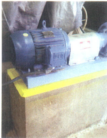
Motor replacement on belt press.
