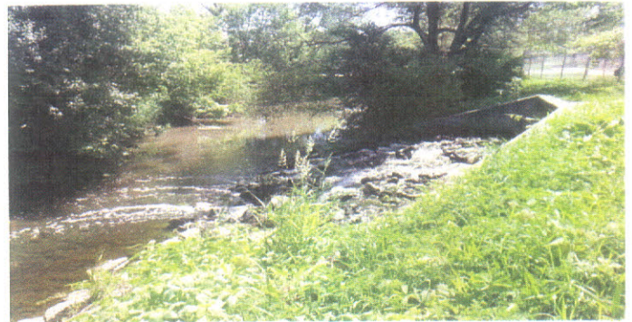
Finished treated effluent to Klein Creek.
