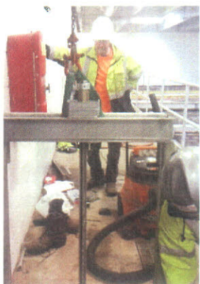
Sand filter gate replacement.
