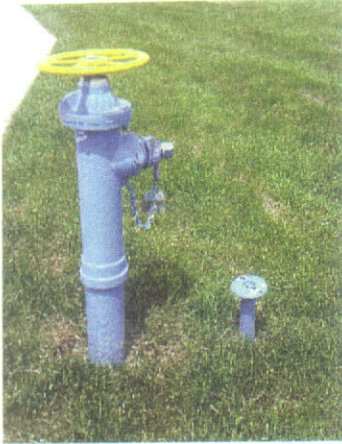
Replacement of yard hydrants.
