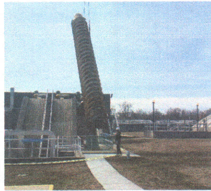
Primary screw pump removal for rehabilitation.
