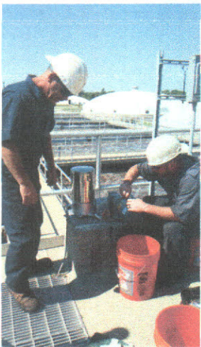
Grease pump installation.
