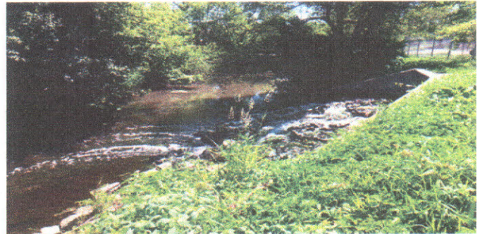
Finished treated effluent to Klein Creek.
