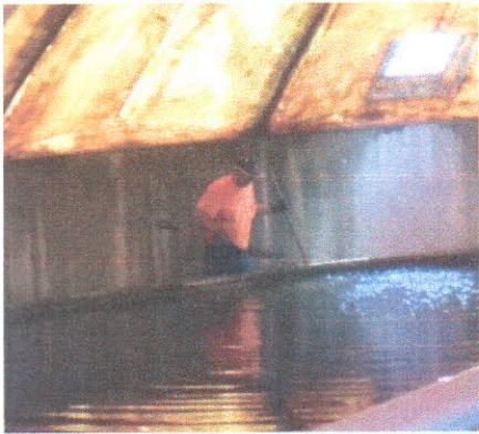
Clarifier cleaning in progress.
