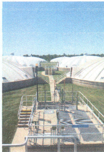
Overview of RAS/WAS station.
