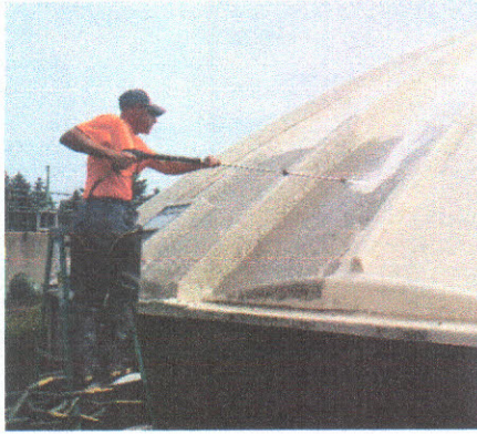
Power washing domes.
