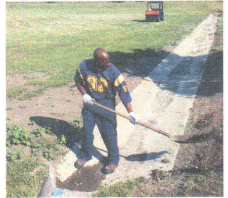
Storm drainage restoration.
