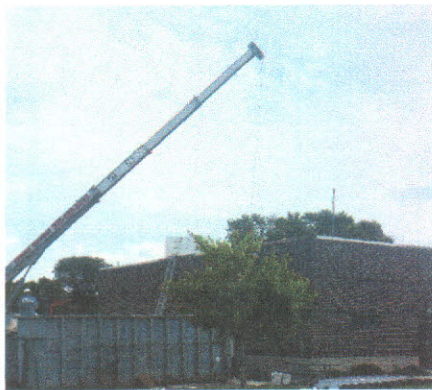
Administration building new roof.
